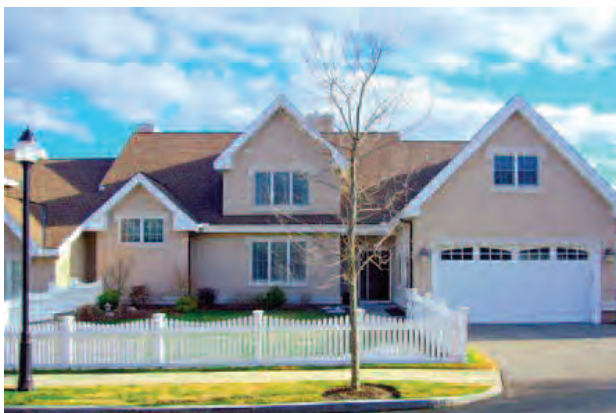
287 Langley Road, 3 Units
